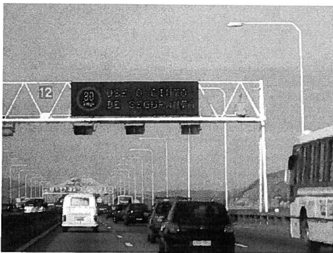
FIGURE 63.3. A changeable-message highway sign in Rio de Janeiro, Brazil. (See Color Plate 23).
