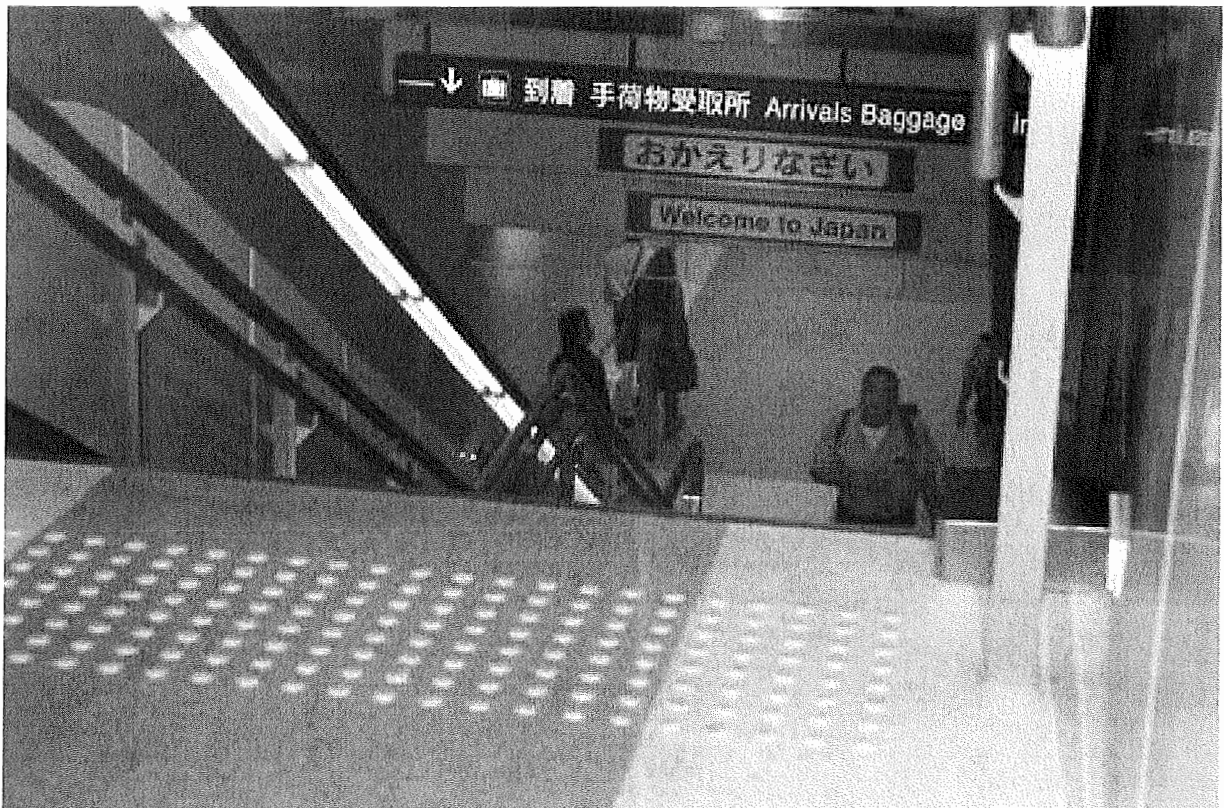
FIGURE 9.3. Detectable tactile warnings at the edge of descending stairs in a Japanese airport. Reprinted with permission from the Wisconsin Department of Transportation.
